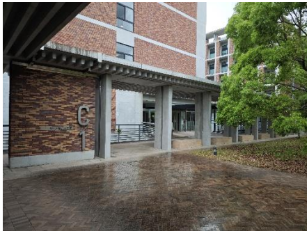
Department of Civil and Earth Resources Engineering: Secretariat of 2024 APSS (No.21 on the map)
